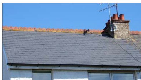
Fig. 22: Slate roofing material
