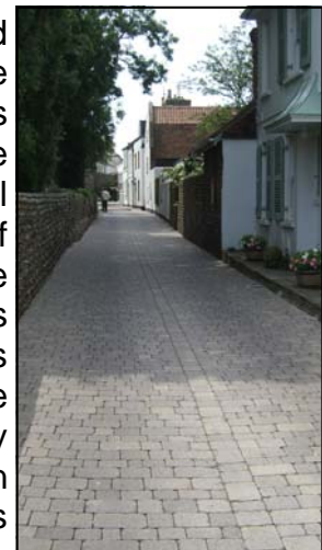
Fig. 34: Tegula Paving in Church Street
