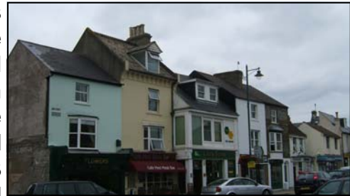
Fig. 18: Roof Variation in High Street
