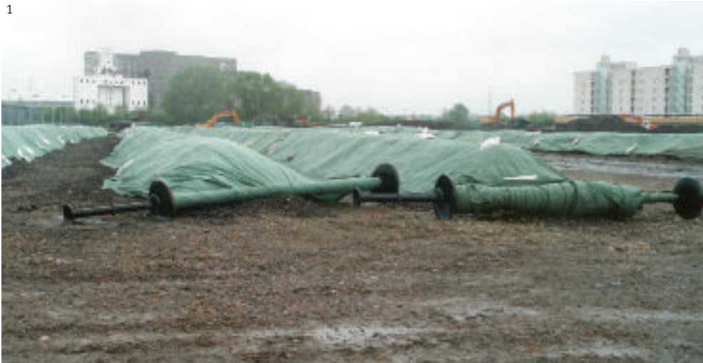
1. On-site remediation using biopiles at an oil refinery.
