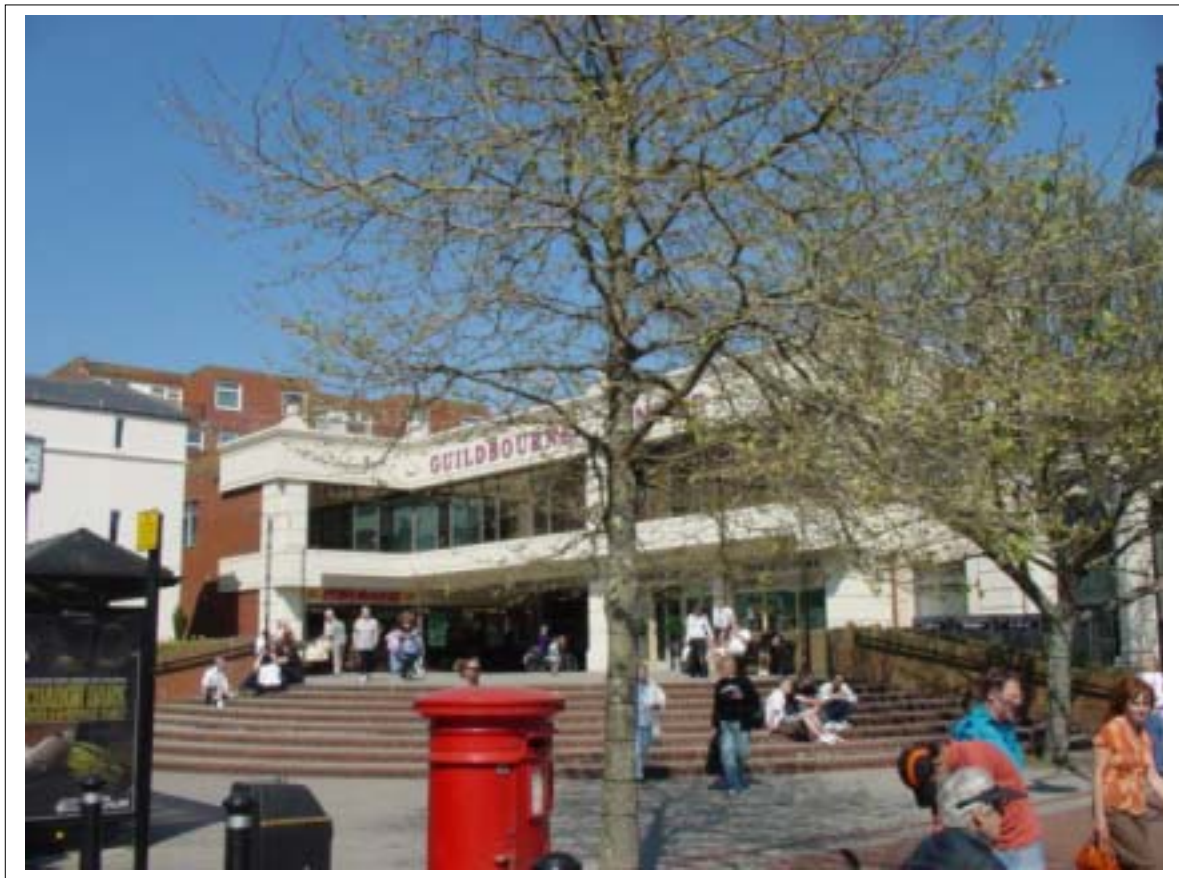
Fig 3.7 Entrance to Guildbourne Centre
