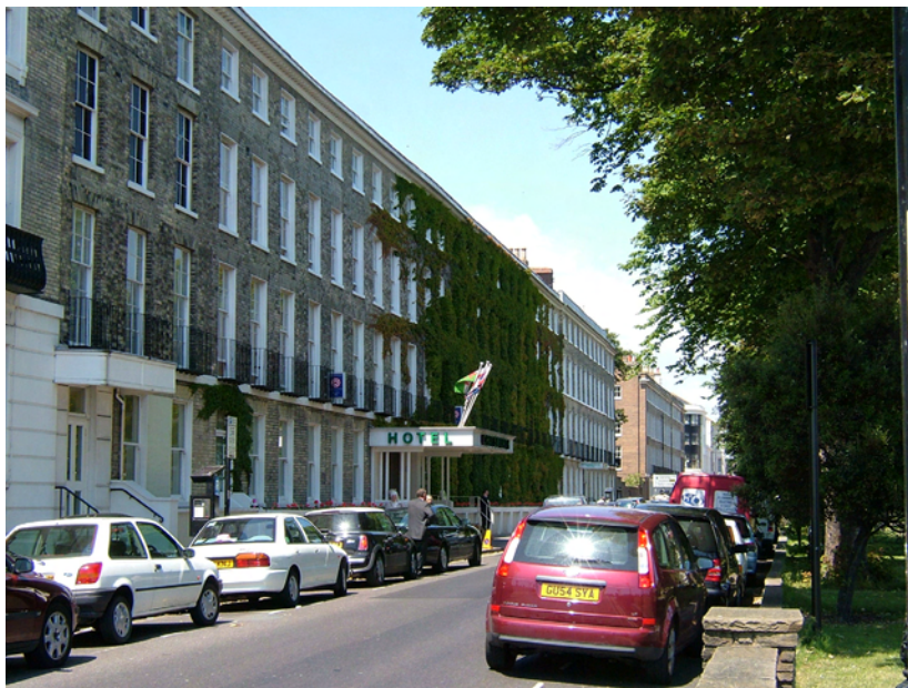
Existing hotel accommodation: Chatsworth Hotel
