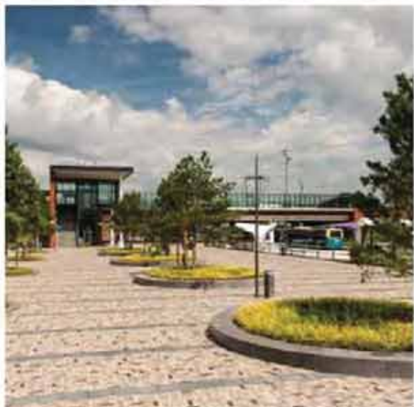
Wider resurfaced paving
