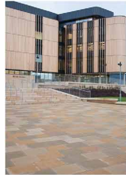
Charcon StoneMaster paving
