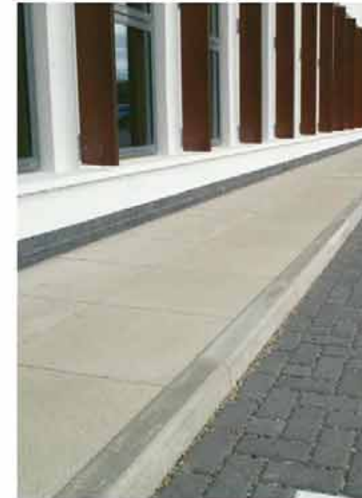
Pre-cast Kerb, St Peter's Square in Manchester
