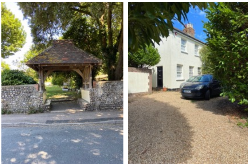
Fig 15: Lych gate to burial ground (left) and 19 th century cottages on St Julian's Lane (right)
