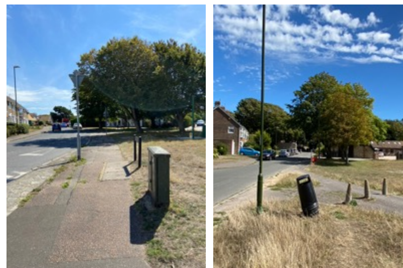
Fig 32: poor quality street furniture and surfaces along St Julian's Lane
