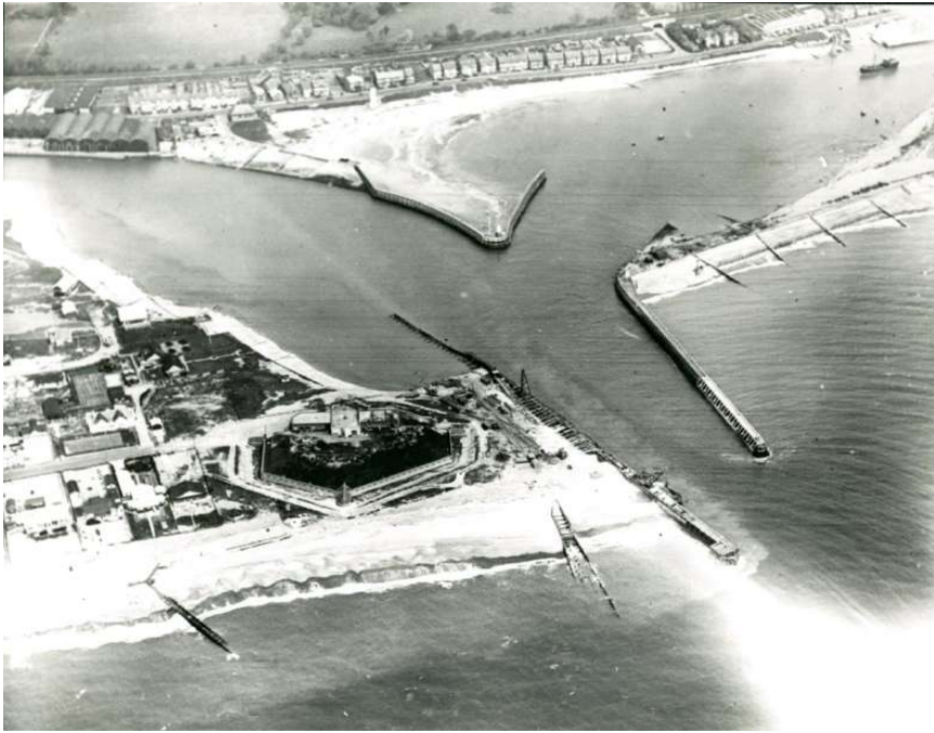
Fig 24: Aerial photograph of Shoreham Port, c1930, Shoreham Fort west of the harbour mouth
