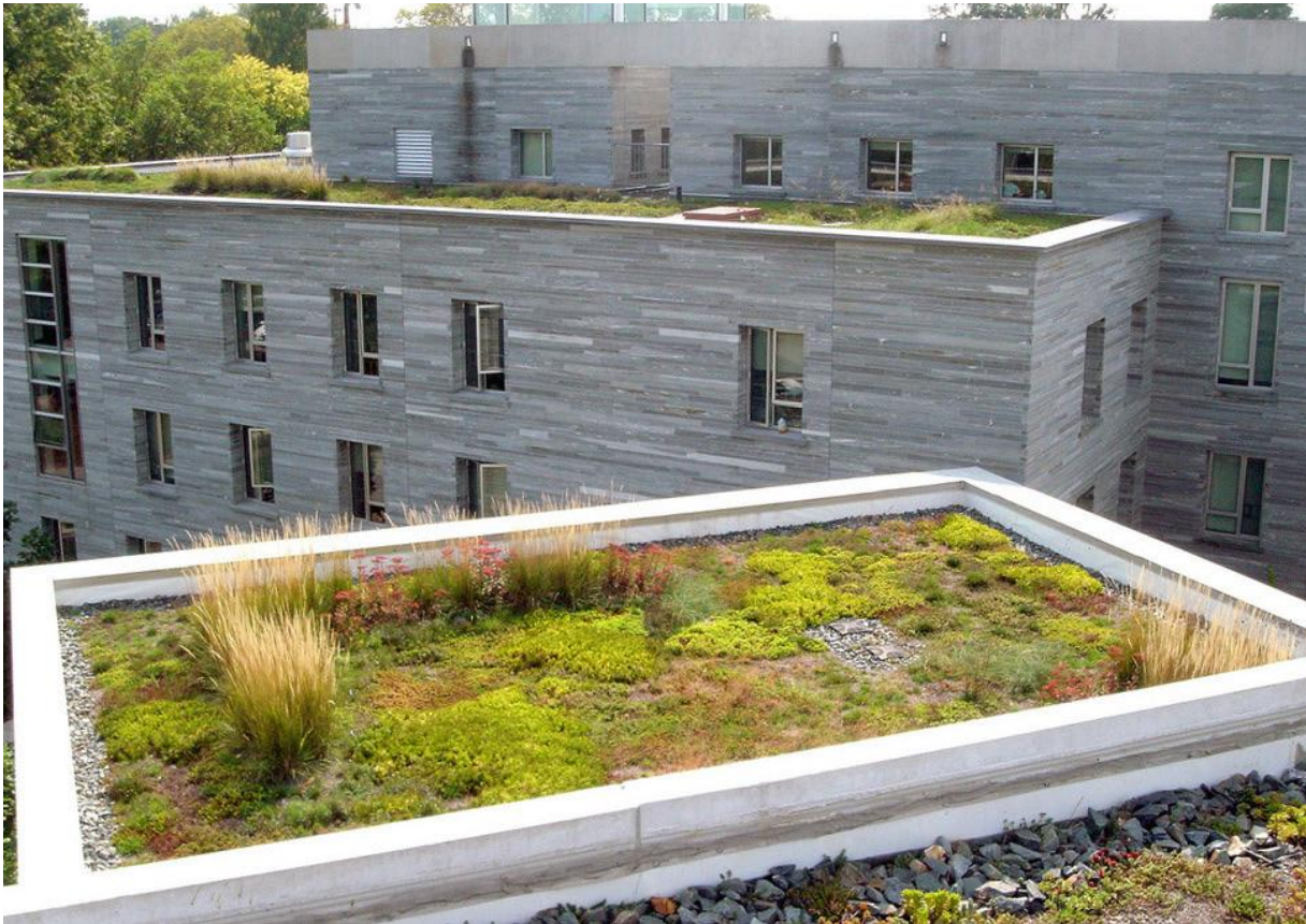
Figure 3.9: Wildflower and sedum green roof 49
