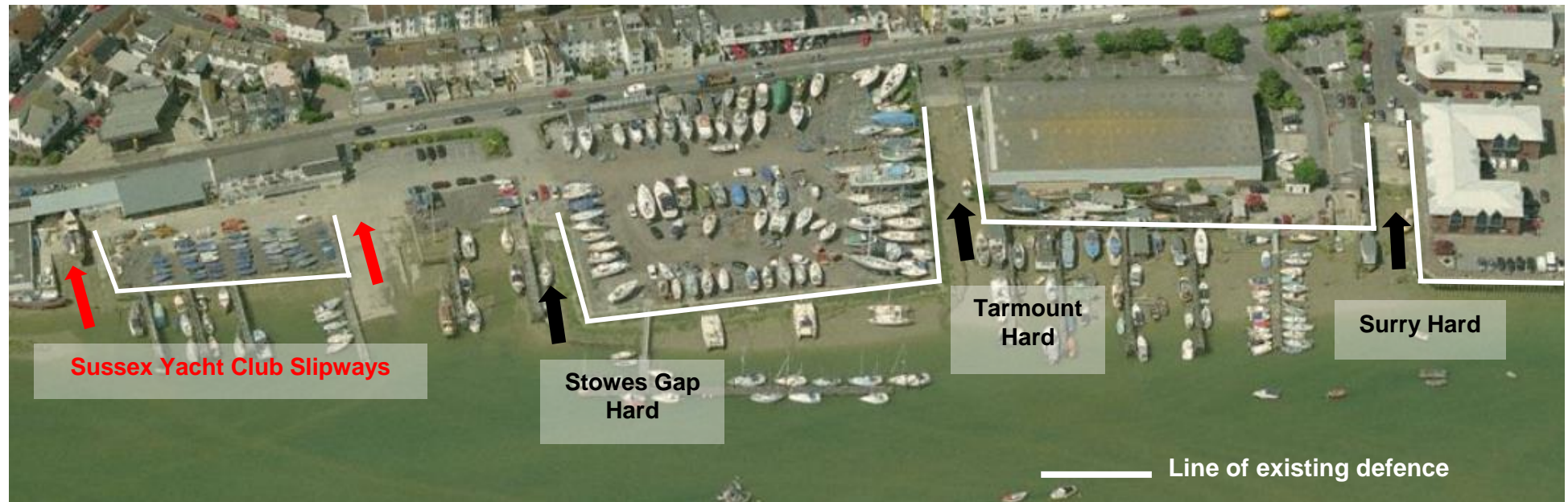
Figure 7.4: Adur Ferry Bridge to Riverside Business Centre - existing defences
