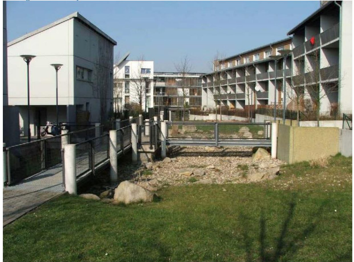
Figure 3.10: Example of sustainable drainage in Germany 55
