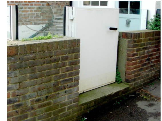
Figure 3.2: Flood door and glazed screen 36
