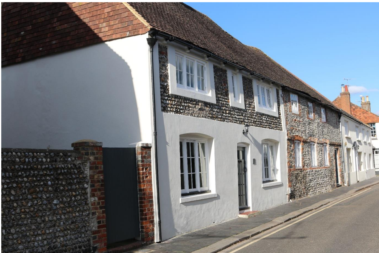
Malthouse Cottage, 3 High Street, Tarring (Grade II Listed)
