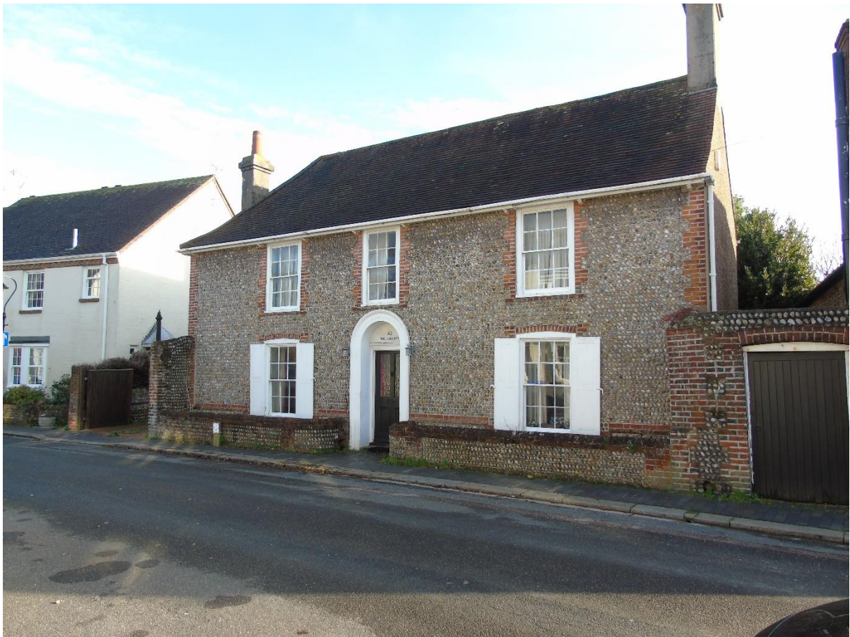
The Hollies, 42 High Street, Tarring. (Grade II Listed)
