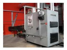
Figure 45 - communal biomass boiler
