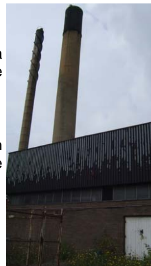
Fig. 25: Boiler house and chimneys
