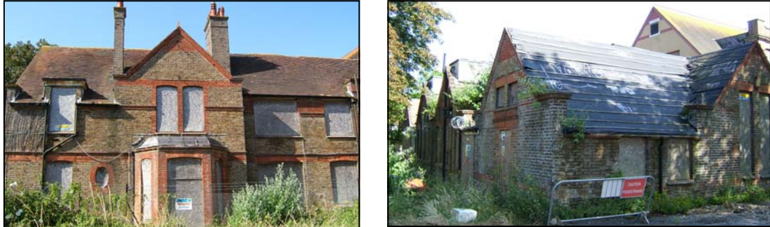
Figs. 12 & 13: Secondary halls (south elevation) and kitchen block
