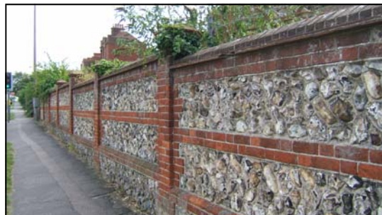
Fig. 21: Front boundary wall
