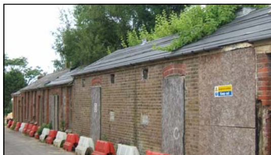
Fig. 4 Accessory buildings on site
