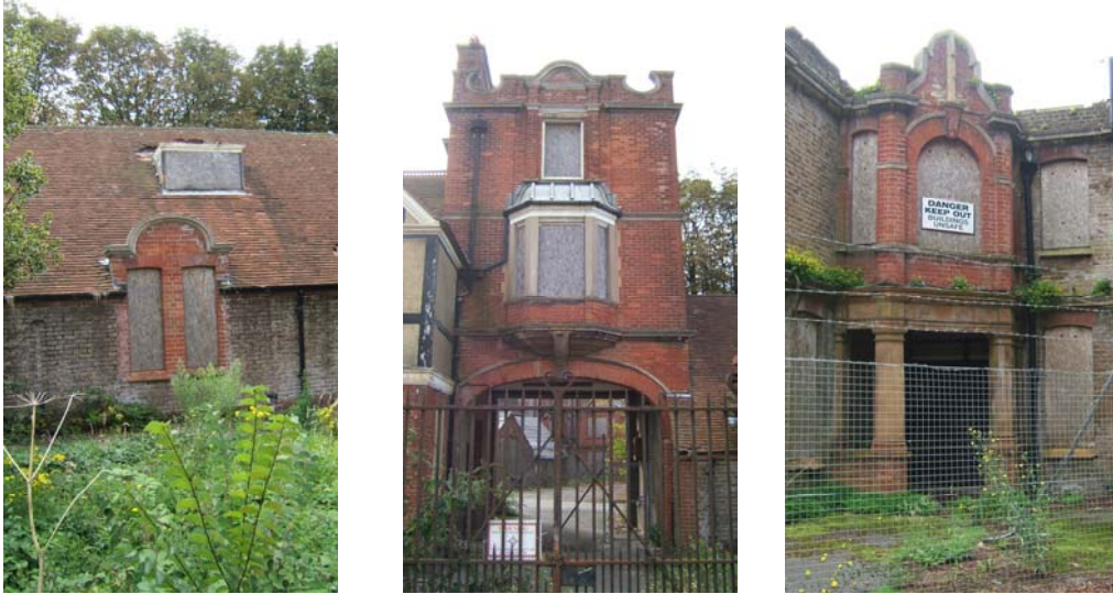
Figs. 5, 6, 7: Architectural details (from left): Dutch gable on entrance block, entrance arch on entrance block, entrance to refectory block
