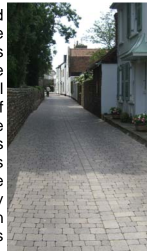
Fig. 34: Tegula Paving in Church Street
