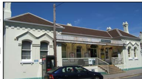
Fig. 30: Shoreham Railway Station
