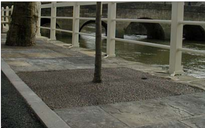
Figure 31. Typical resin bound tree pit
