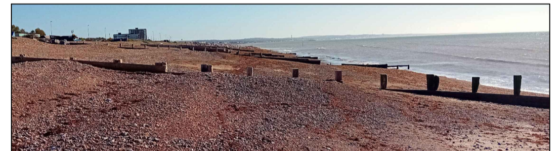
Photo of the same groyne two months after the works were completed
