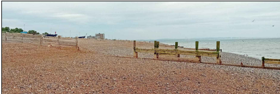
Photo of a groyne before works
