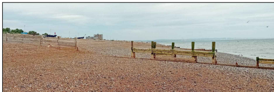
Photo of a groyne before works
