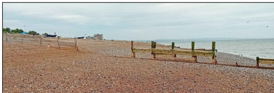
Photo of a groyne before works
