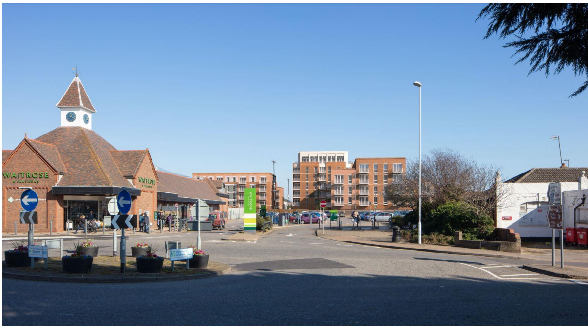
Figure 8: Representative view of site through Waitrose car park (Credit: St William Homes LLP)
