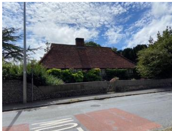
Fig 24: Close-boarded fence over reduced flint wall
