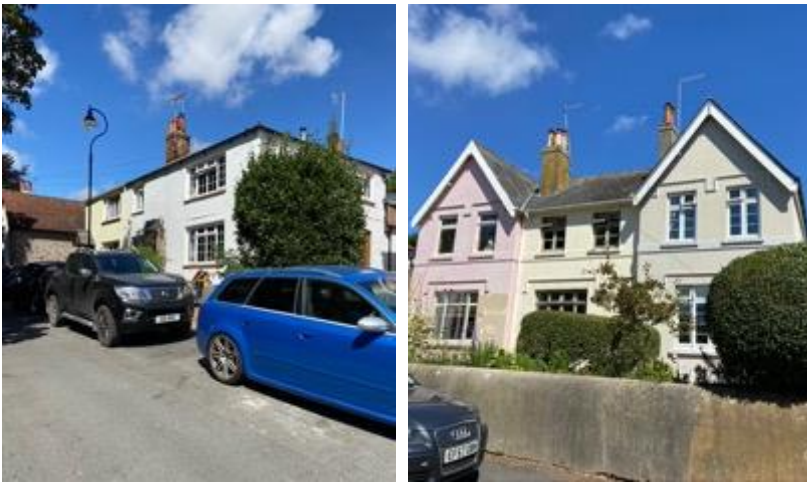
Fig 42: Modern uPVC windows to unlisted historic buildings
