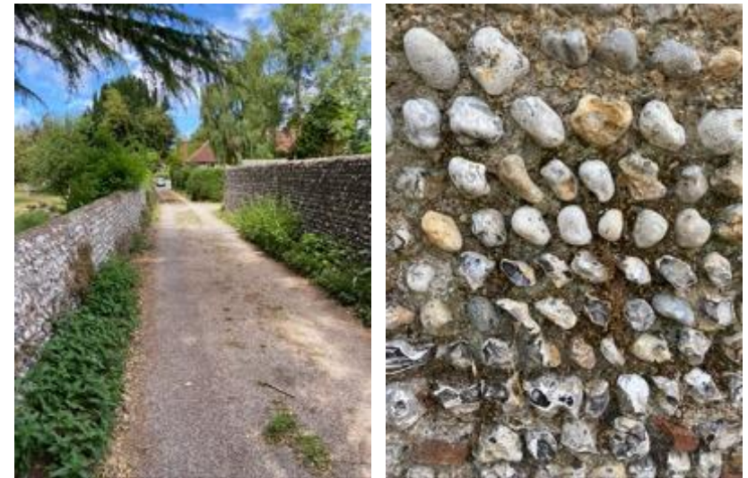
Fig 22: Historic flint walls
