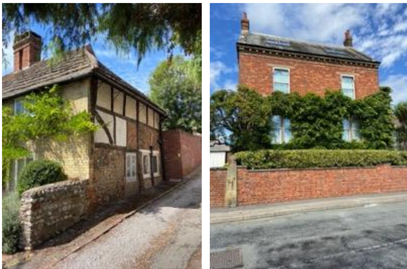
Fig 20: Use of brick in the conservation area, Horsham slab to roof of Grant's Manor
