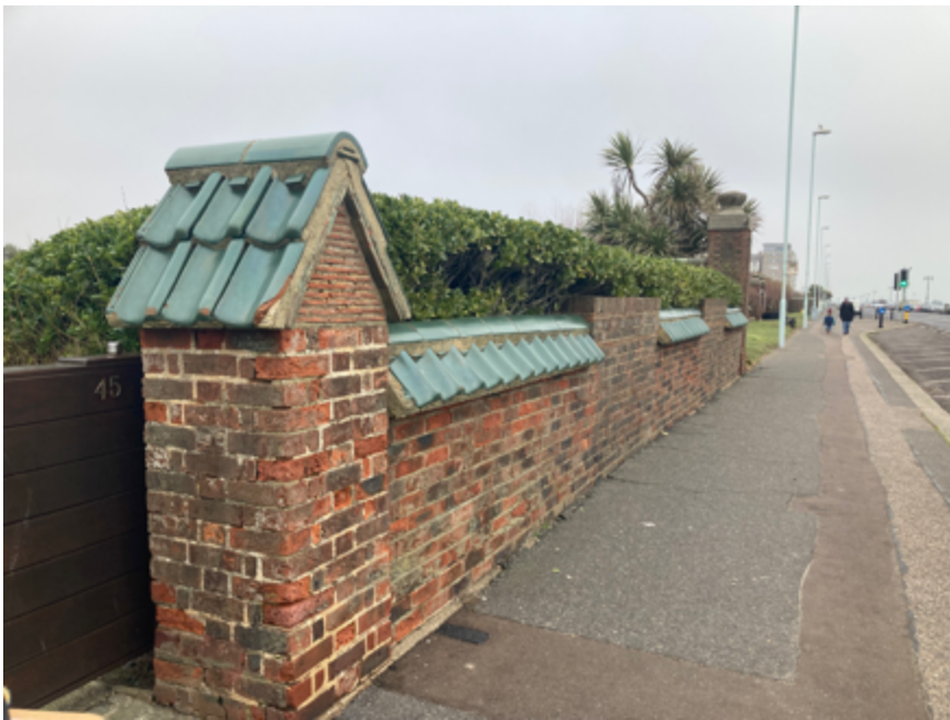
Figure 16: Brick boundary walls with green pantile capping
