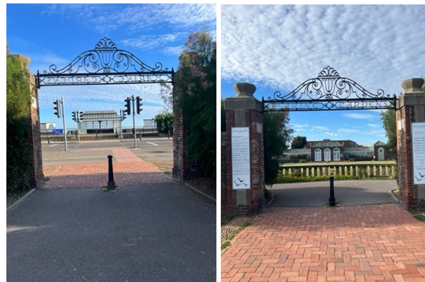
Figure 36: View north and south from entrance gates
