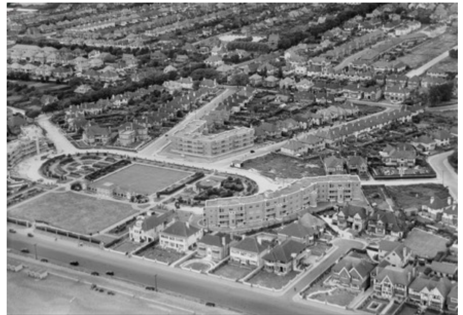
Figure 12: Marine Gardens, view from the south; 1937; Source: Historic England
