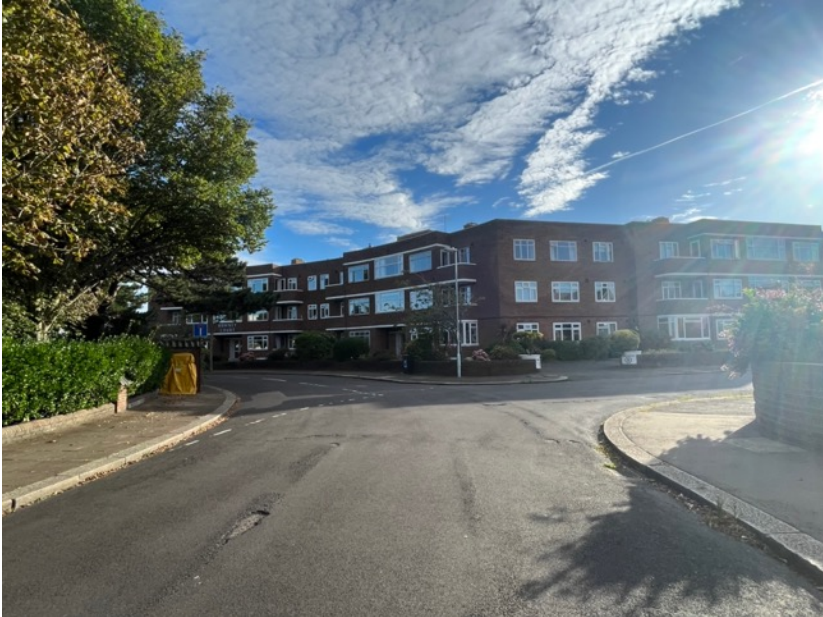
Figure 41: View towards Romney Court from Winchelsea Gardens
