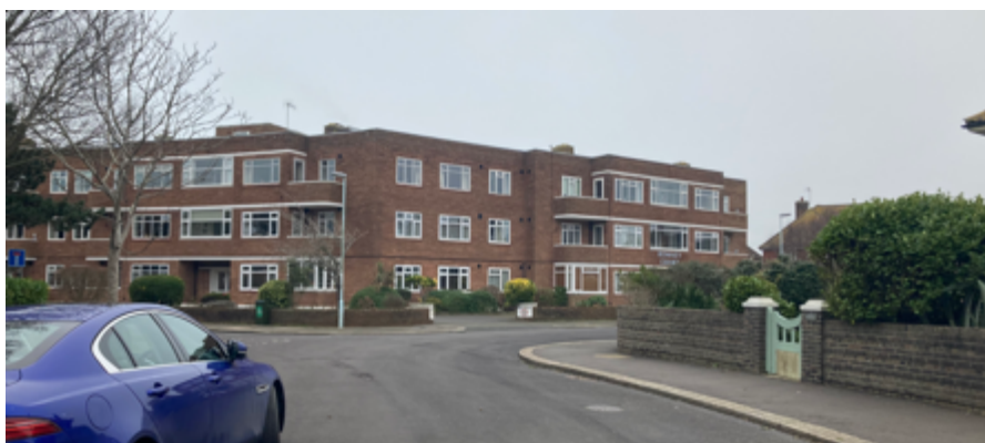
Figure 35: Low brick boundary walls around Winchelsea Gardens
