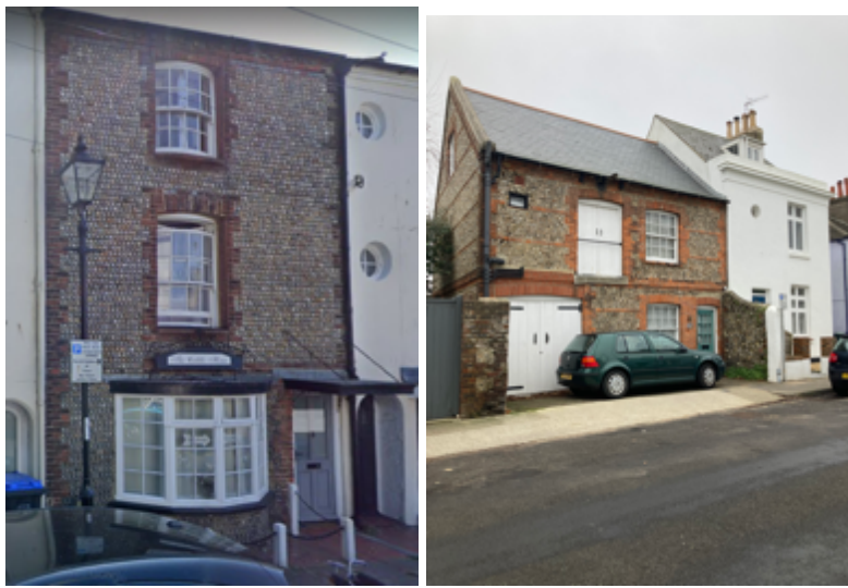
Figure 50: Further examples of flint in the conservation area
