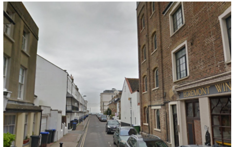
Figure 64: Views south along York Road (top) and Warwick Road (bottom)
