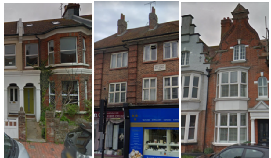
Figure 51: Examples of yellow and red brick in the conservation area
