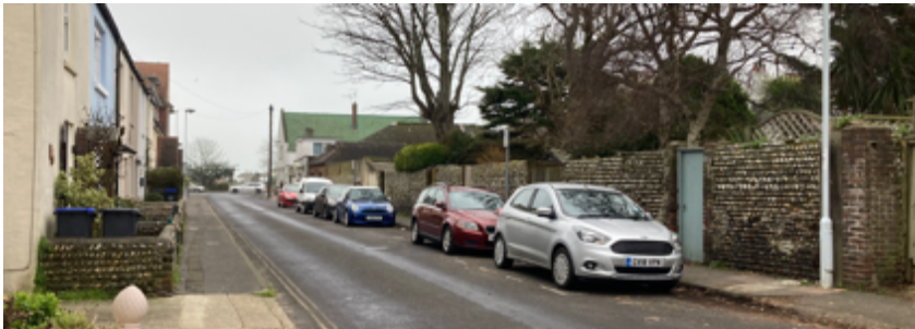
Figure 53: Examples of boundary walls and railings
