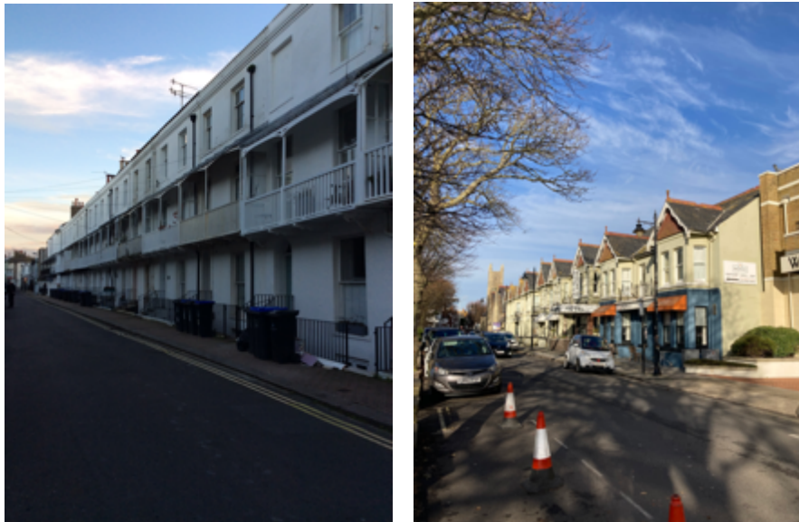
Figure 13: Examples of residential buildings on Warwick Road (left) and Steyne Gardens (right)
