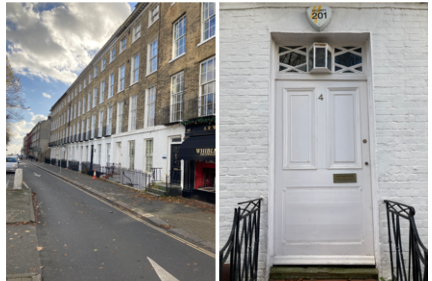
Figure 27: Northern terrace on The Steyne
