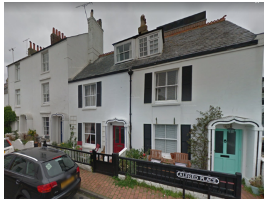
Figure 33: Listed buildings on Alfred Place
