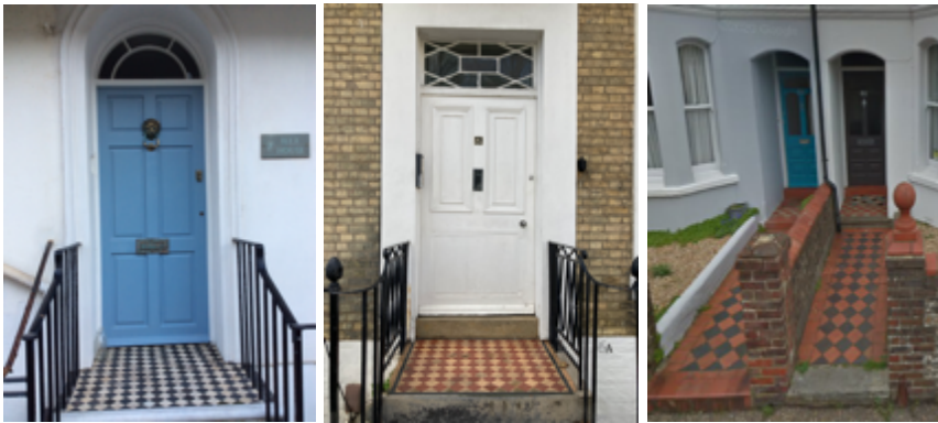
Figure 56: Pavements and tiling within the conservation area
