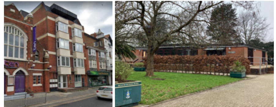
Figure 59: No. 8 High Street and Bowling Club House, Beach House Park
