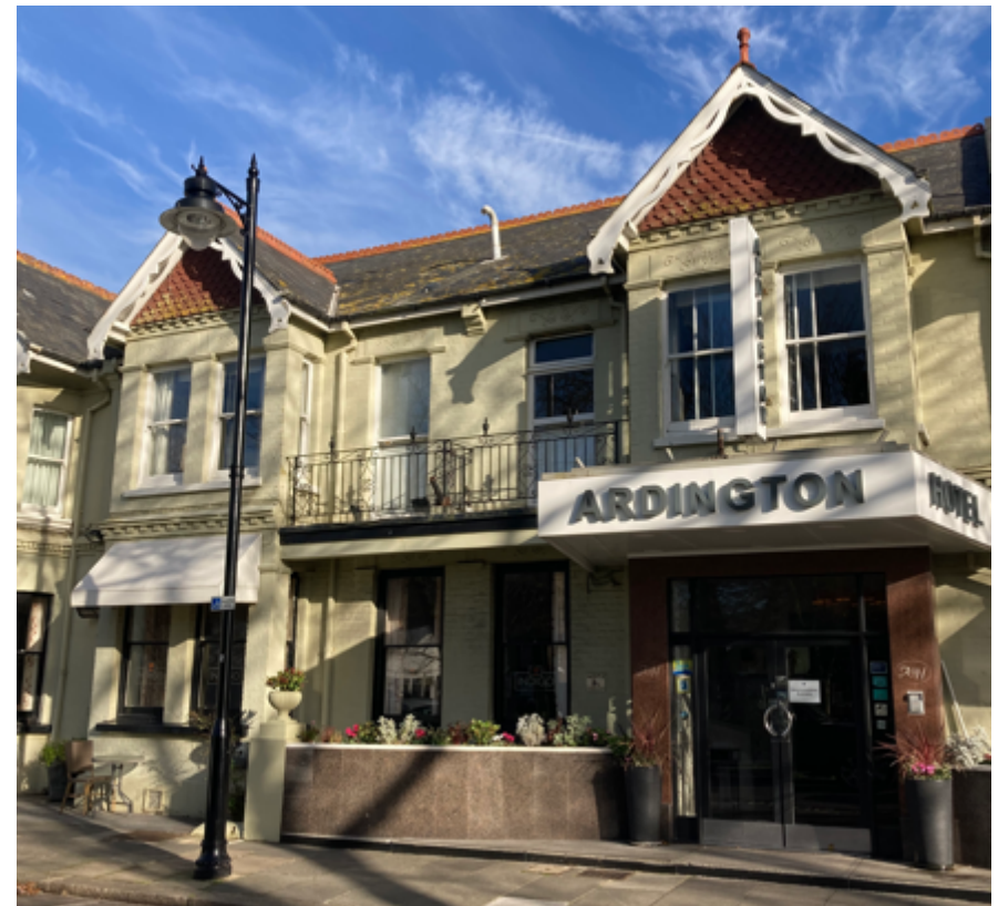
Figure 29: Part of the terrace at 30-38 Steyne Gardens
