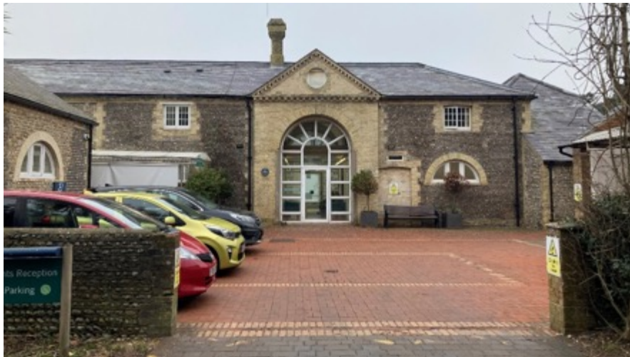
Figure 21: Former stable building at Goring Hall
