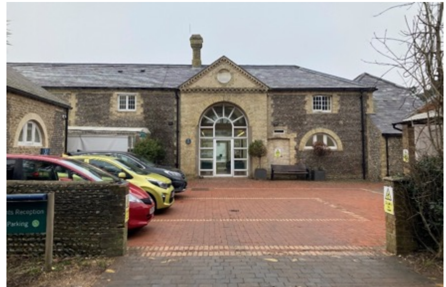
Figure 13: Former Stable building to Goring Hall (listed grade II)
