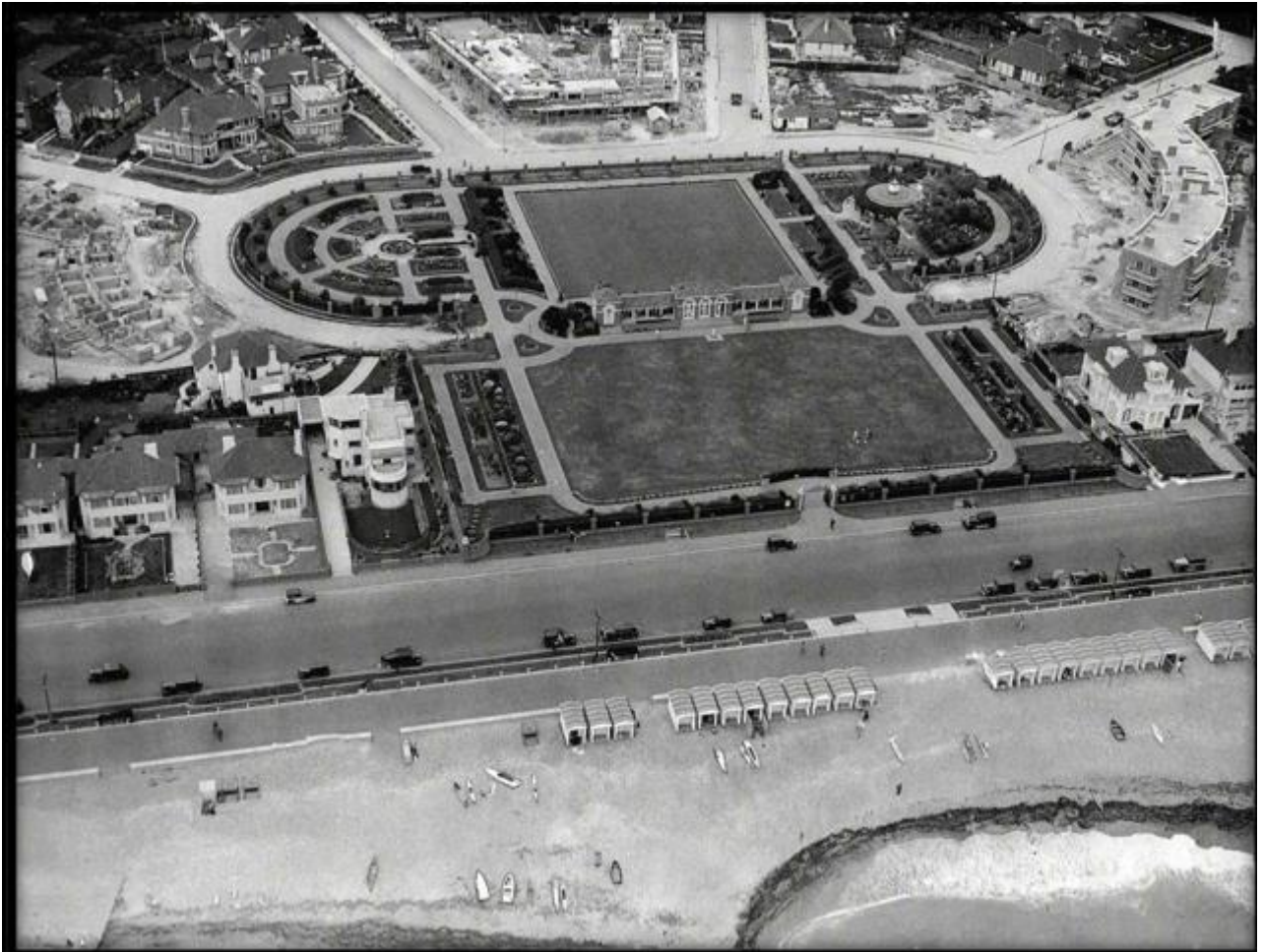
Figure 18: Aerial photograph showing the development of Marine Gardens and the surrounding area
