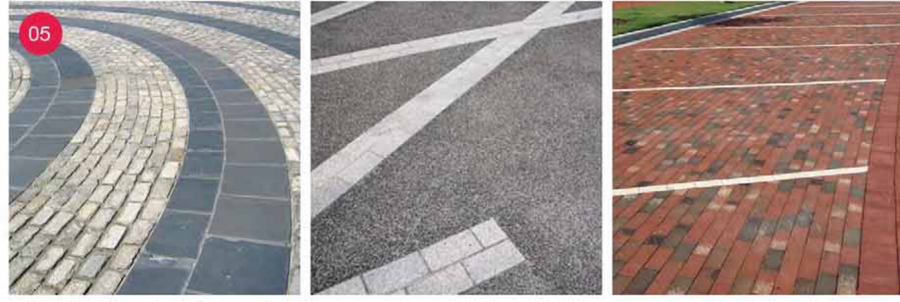
Banding in contrasting paving
