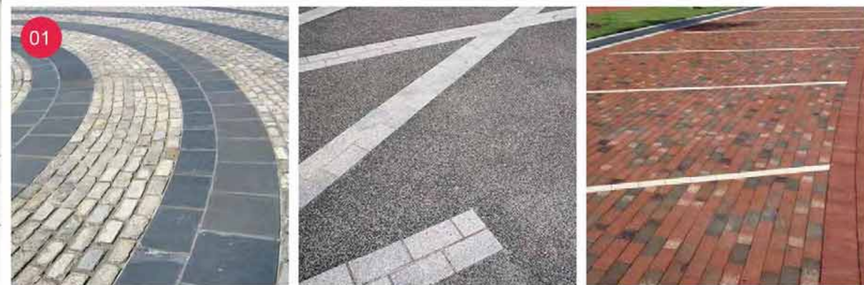
Banding in contrasting paving
