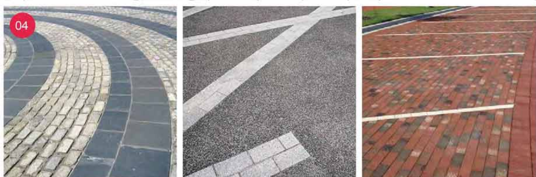
Banding in contrasting paving
