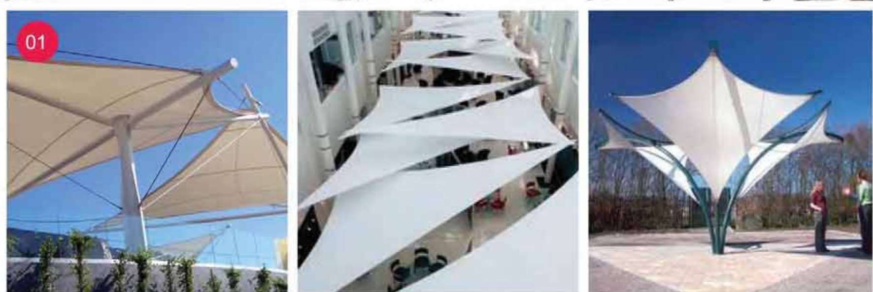
Tensile fabric shade structure
