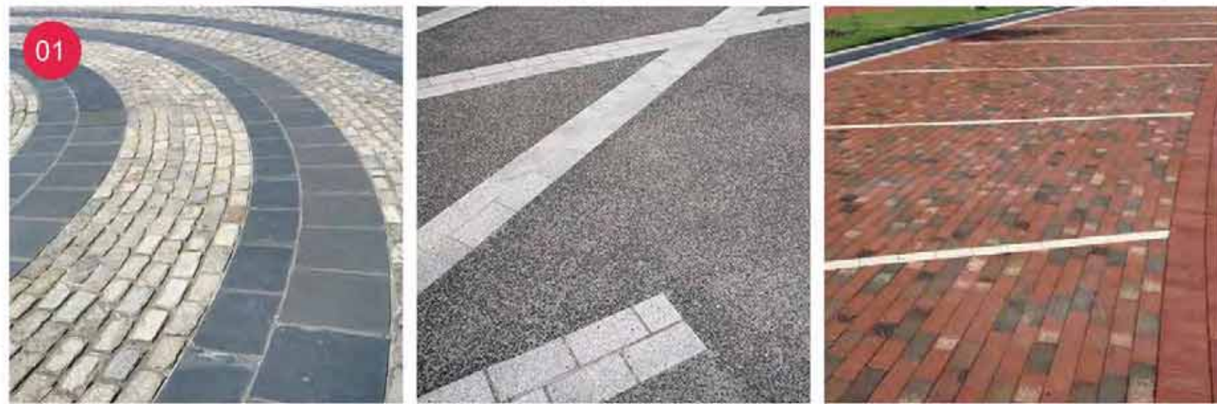
Banding in contrasting paving
