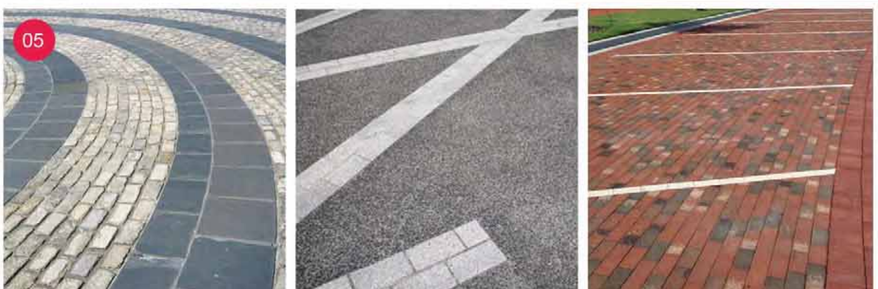
Banding in contrasting paving
