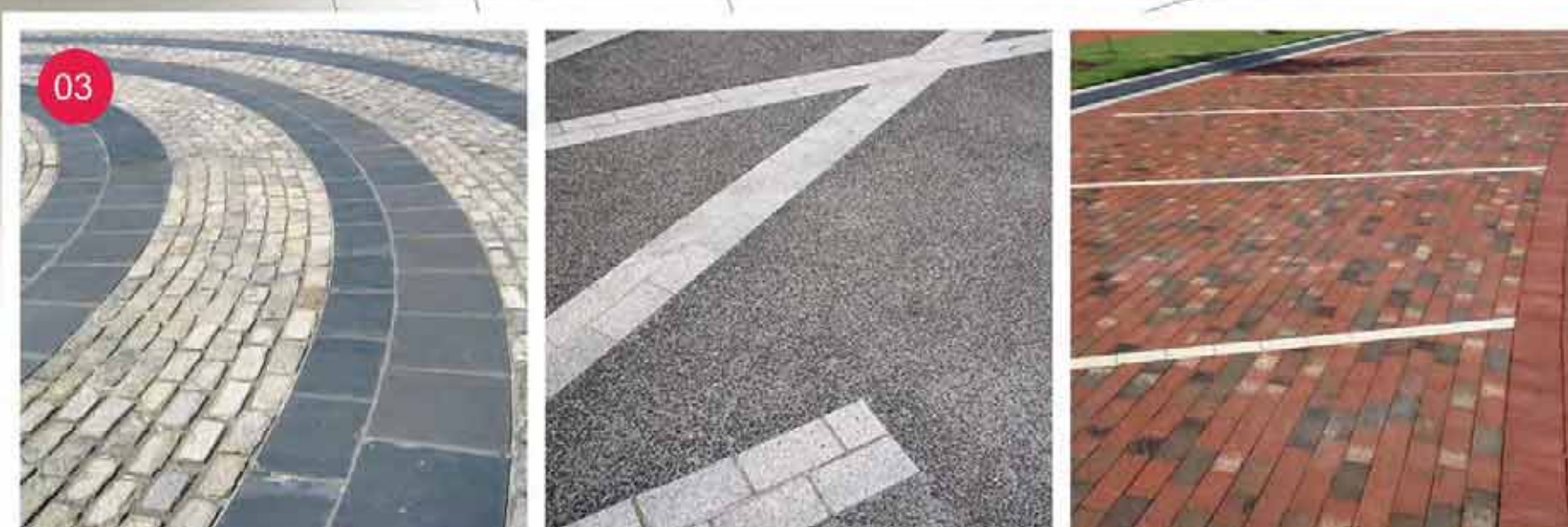
Banding in contrasting paving
