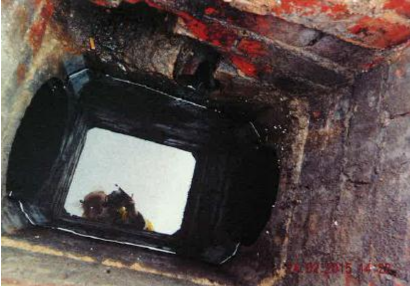
Figure 5-4 Photo of manhole on A259 (taken by WSCC)
