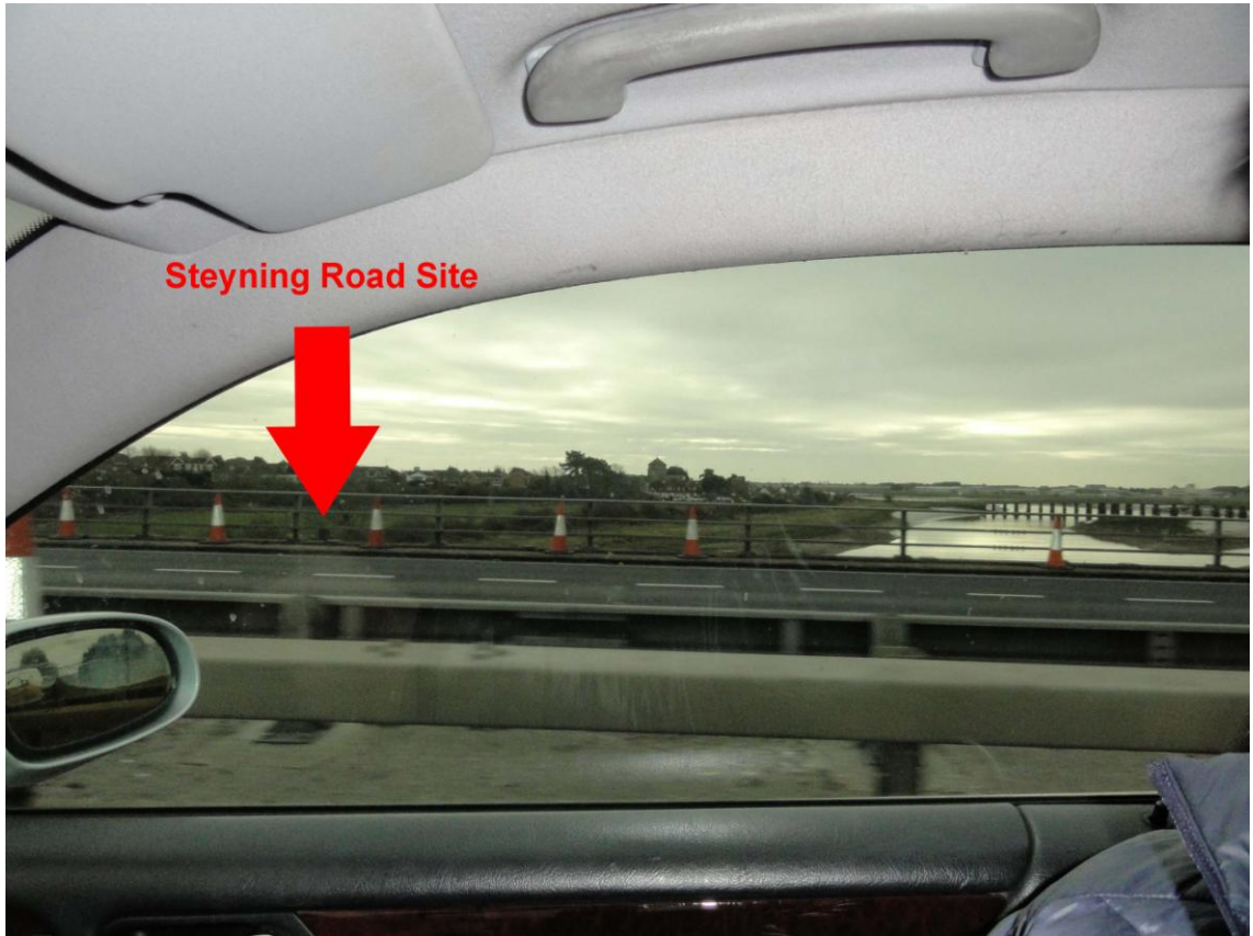
View: South from East bound carriageway of elevated A27 flyover
