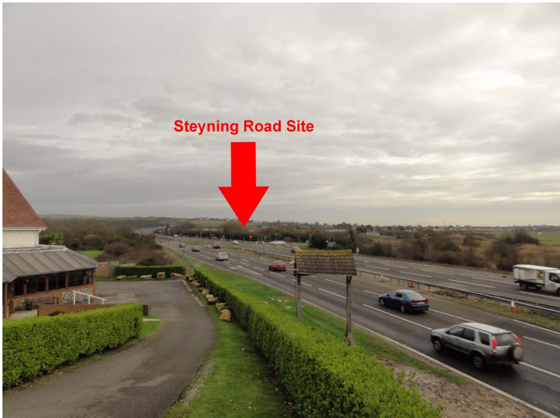
View: East from Sussex Pad showing roof tops of Ricardo's works (Site centre)
