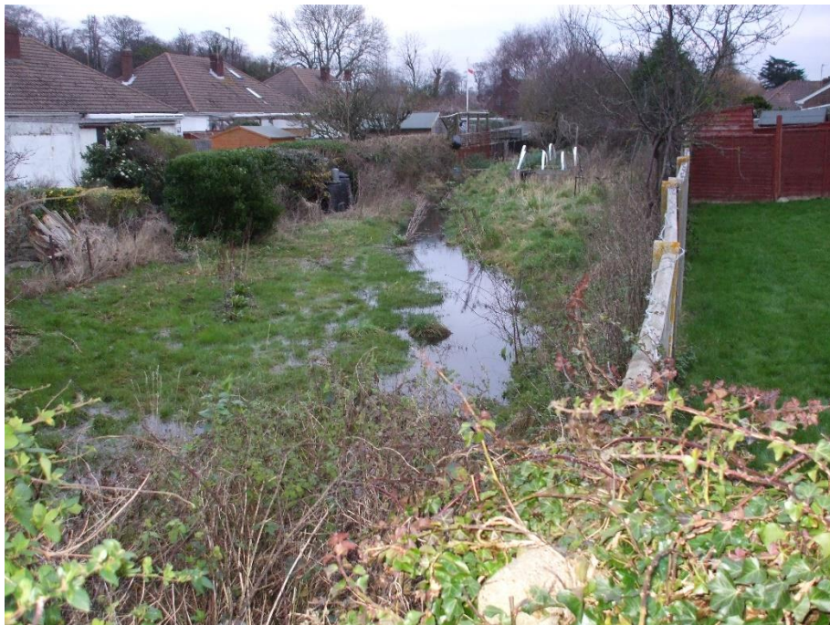
Flooded Ditch behind Old Shoreham Road, 1 January 2013
