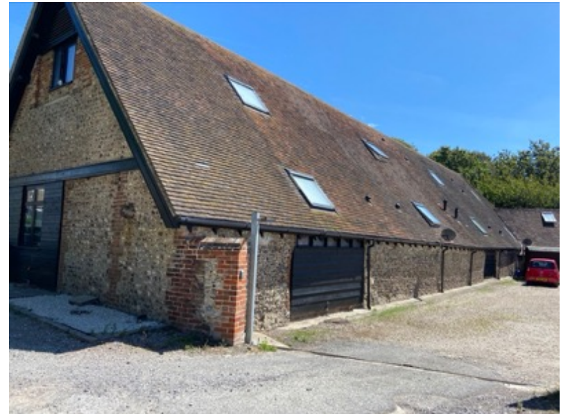
Fig 12: Flint rubblestone and Hythe stone dressings
