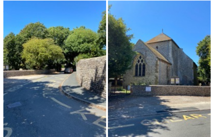
Fig 27: Unfolding view of core of conservation area in approach from the east along St Julian's Lane
