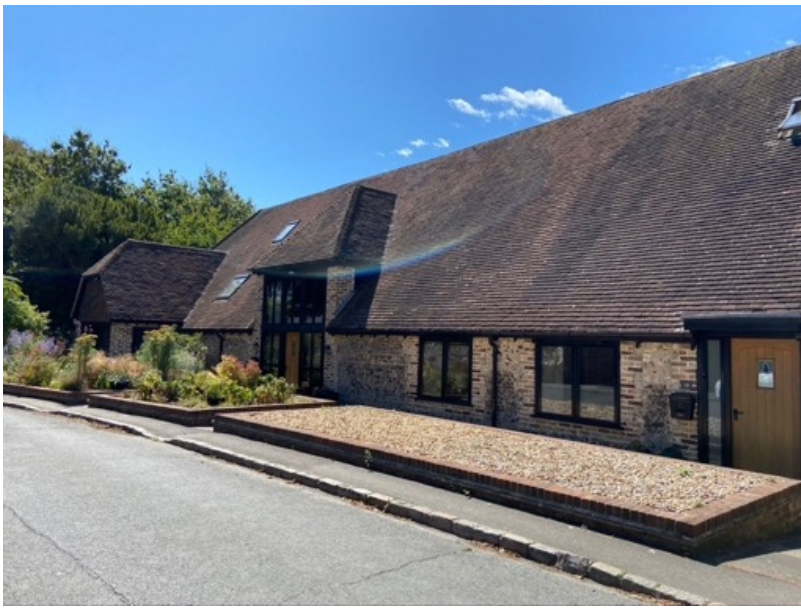
Fig 33: Domestic character of barn and setting
