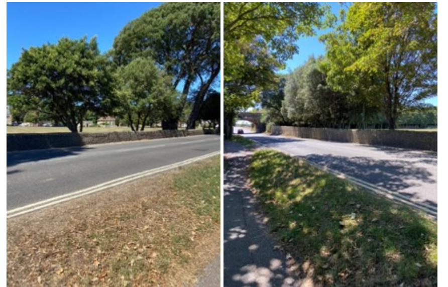
Fig 30: Present day views along Kingston Lane
