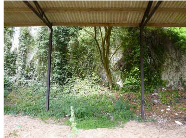
4. Vegetated chalk face at back of third open shed. Grid ref. TQ014820574. Direction west.
