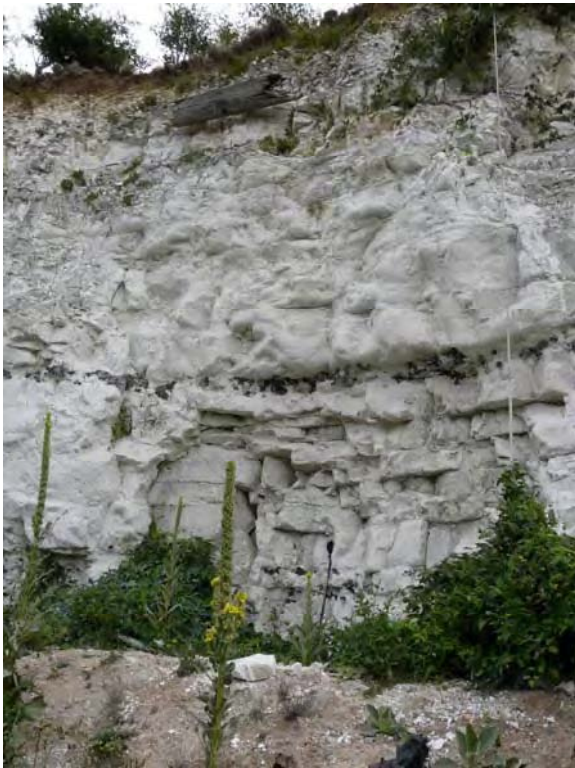
5. Part of central chalk face showing prominent Charmandean Flint band at centre, thinner flint bands near base and possible thin marl seams in the upper section. Face 5.5m high. Grid ref. TQ15640590. Direction east.
