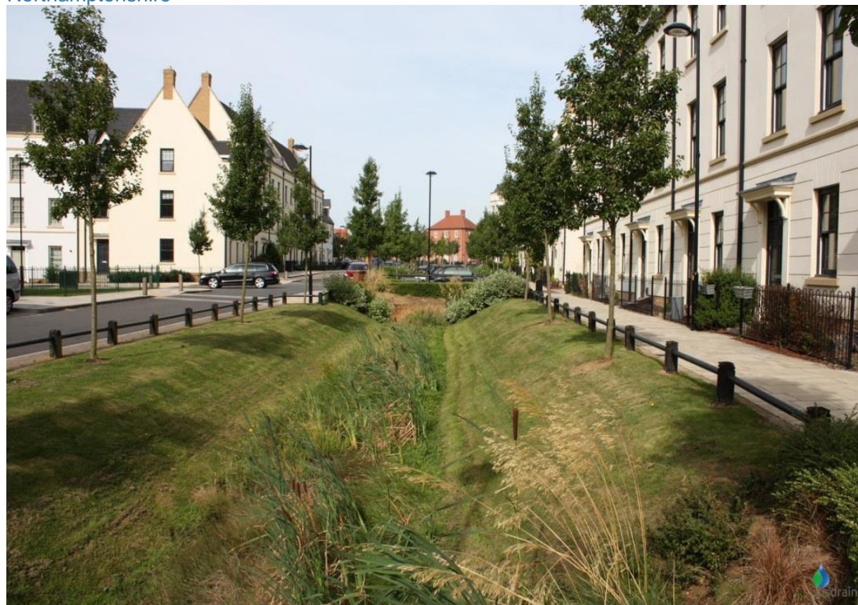
Figure 3.8: Swales at Upton, Northamptonshire 48
