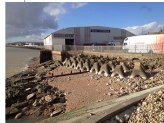
Figure 7.19: Existing defences - concrete revetment 87
