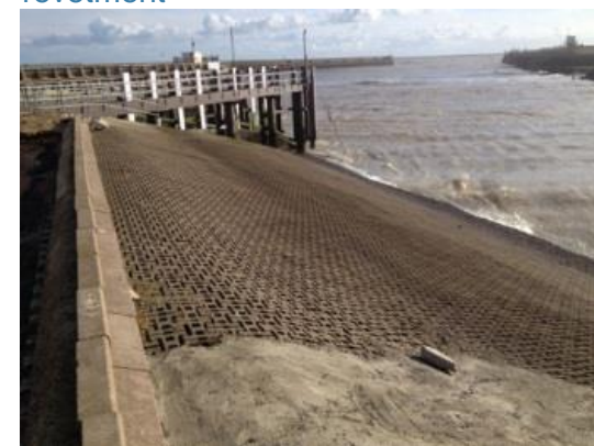
Figure 7.19: Existing defences - concrete revetment 87
