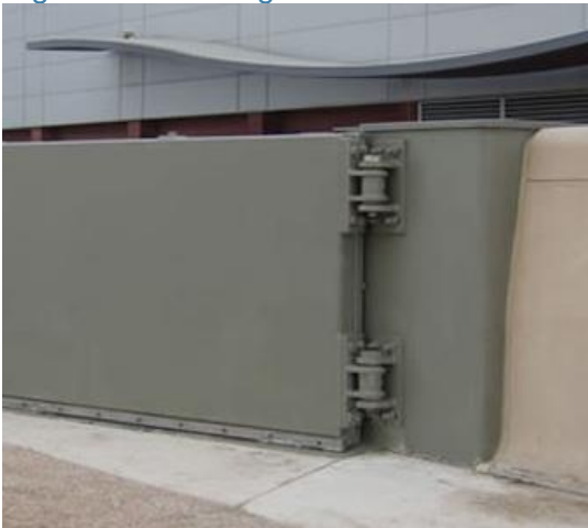
Figure 7.7: Flood gates 72
