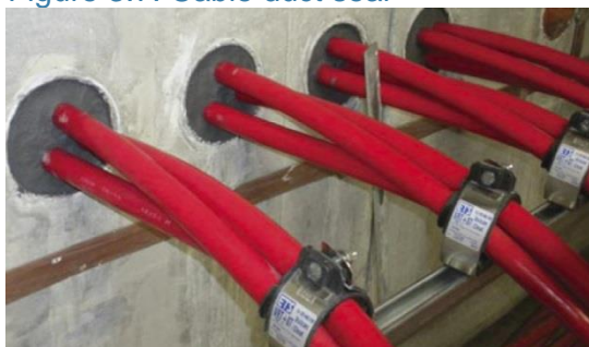
Figure 3.7: Cable duct seal 41
