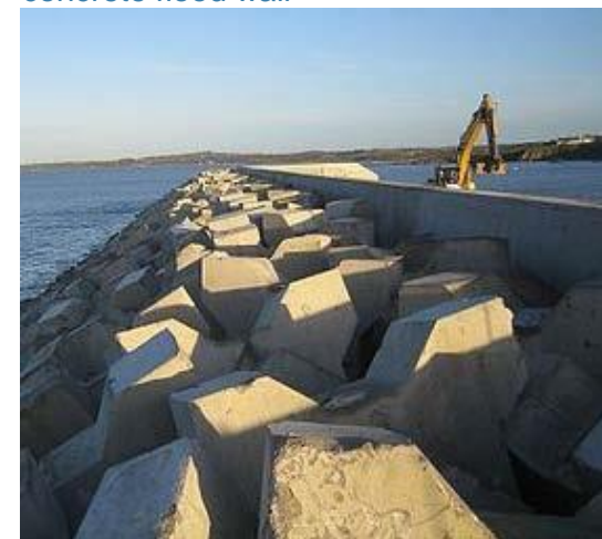
Figure 7.23: Rock revetment with concrete flood wall 91
