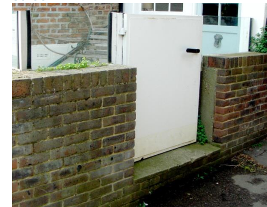
Figure 3.2: Flood door and glazed screen 36
