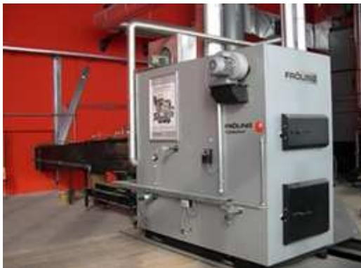
Figure 45 – communal biomass boiler
