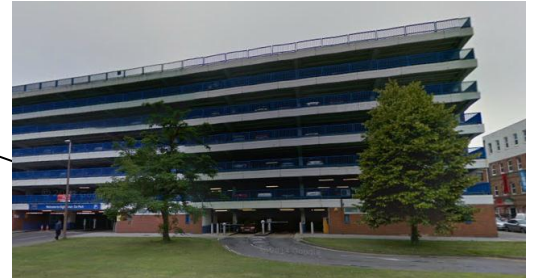
Town Centre Car Park (High Street)
