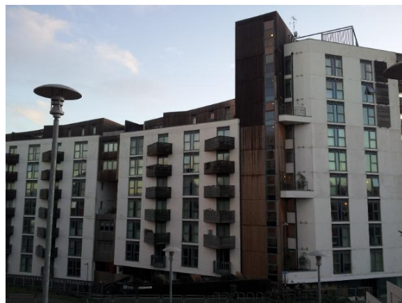
Figure 7. A cluster of tall buildings to the rear of Brighton Station on Stroudley Road, which have contributed positively to the regeneration of this area.
